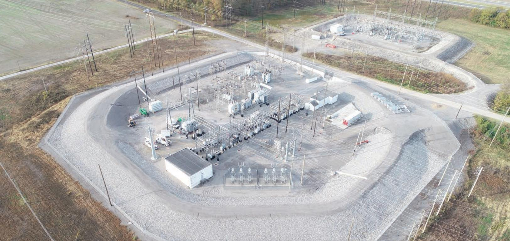
Example of enhanced berm at an Ameren substation for additional flood protection.
